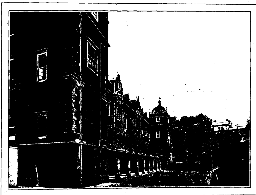
THE CLOISTERS, OLD BLUECOAT SCHOOL, NOW USED AS NURSES' HOME, ST. BARTHOLOMEW'S HOSPITAL, LONDON, E.C.
